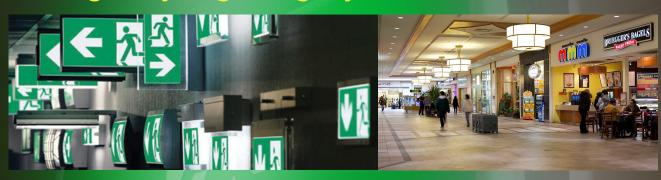
The purpose of emergency lighting is to ensure the lighting is provided promptly, automatically and for a suitable time when the normal power supply to the lighting fails to ensure that people within the building can evacuate safely in the event of an emergency. Emergency lighting can be provided by means of local self-contained batteries mounted within the emergency luminaire or by a central battery wired via a dedicated network to the emergency fittings.
